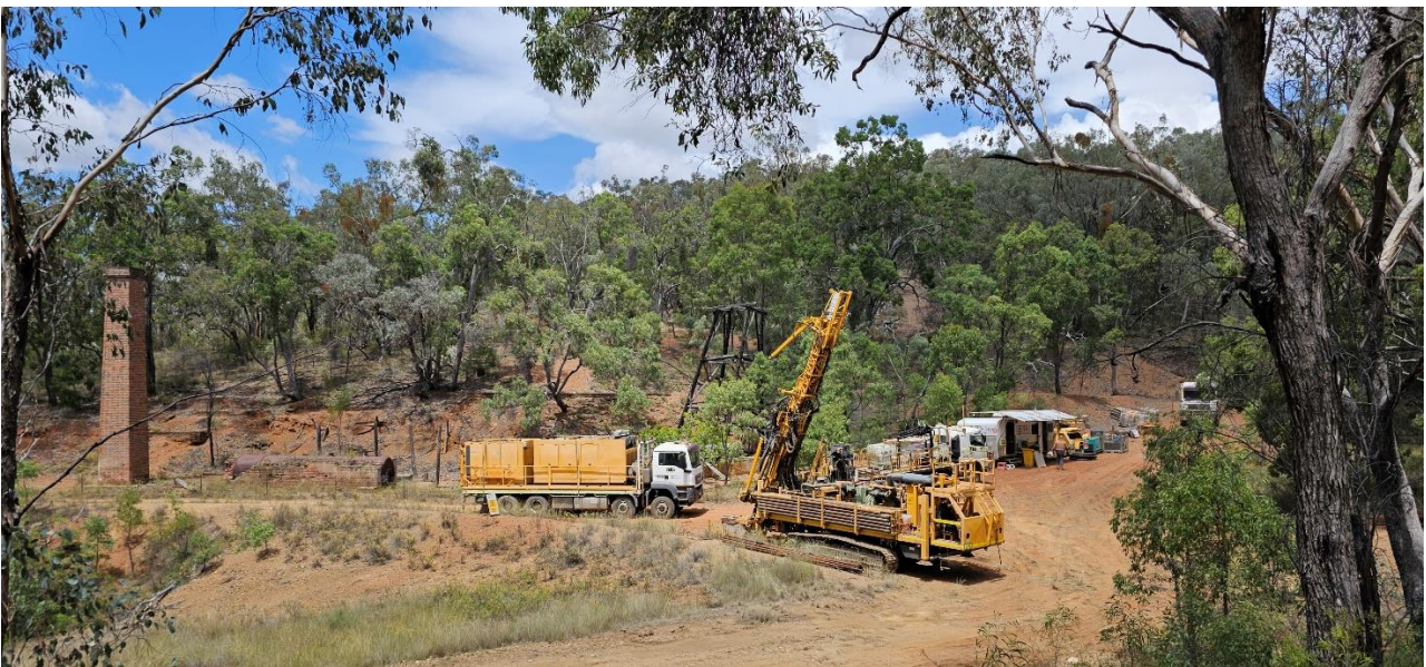
Figure 1: Drilling Equipment located next to the old Gulf Creek Copper Mine headframe and smelter stack
